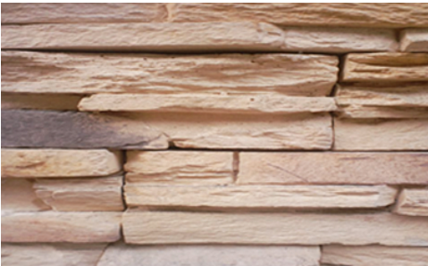
Figure 5.17 An example of a complex wall surface
